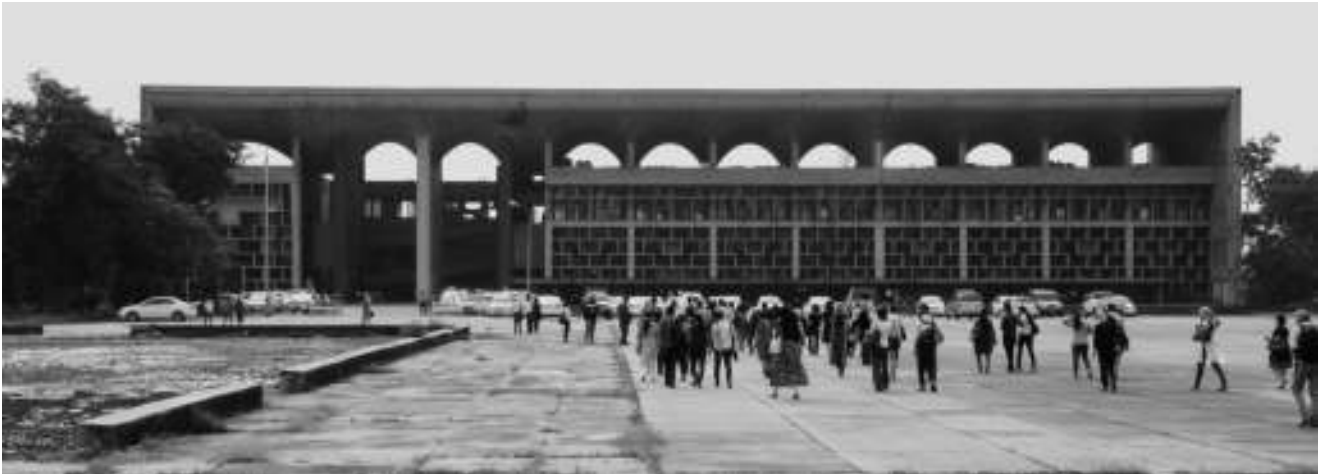
01-03 Le Corbusier, Capitol Complex, Chandigarh, India, 1962. © Ana Tostões, 2013.
